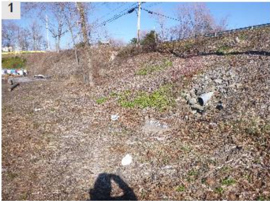
Upper parking area existing outfall pipe.
