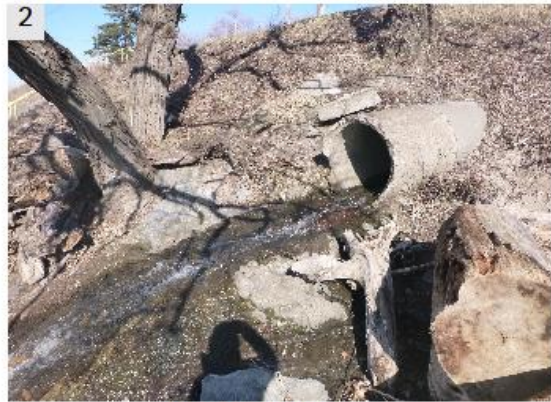
Existing beach outfall pipe.
