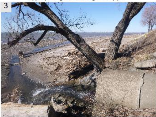
Existing beach outfall pipe.
